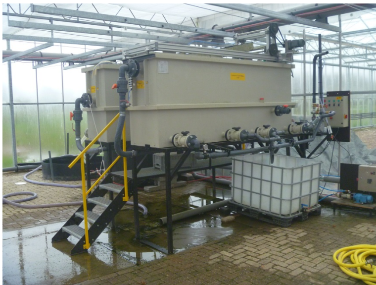
Figure 31. Dissolved air flotation unit.
