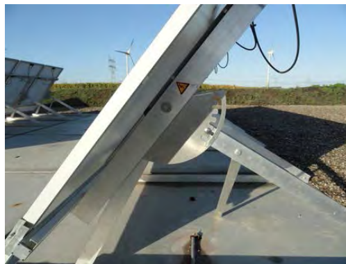
Foto 6: variabele opstelling (Schletter Vario Top)
